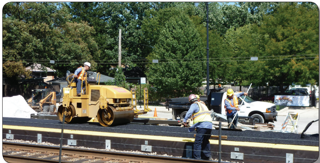
Workers resurface the platform at the Edgebrook Station on the Milwaukee North Line.
