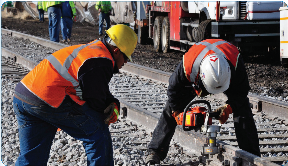
Metra signal maintainers apply a bond wire to a join in the rail.
