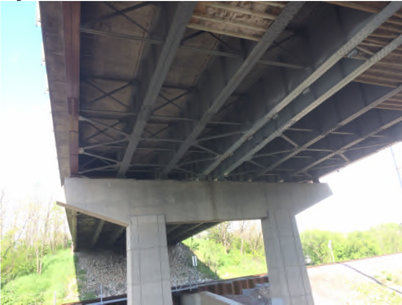
Photo 7: Representative photograph from under the U.S. Route 20 Bridge over the Fox River.
