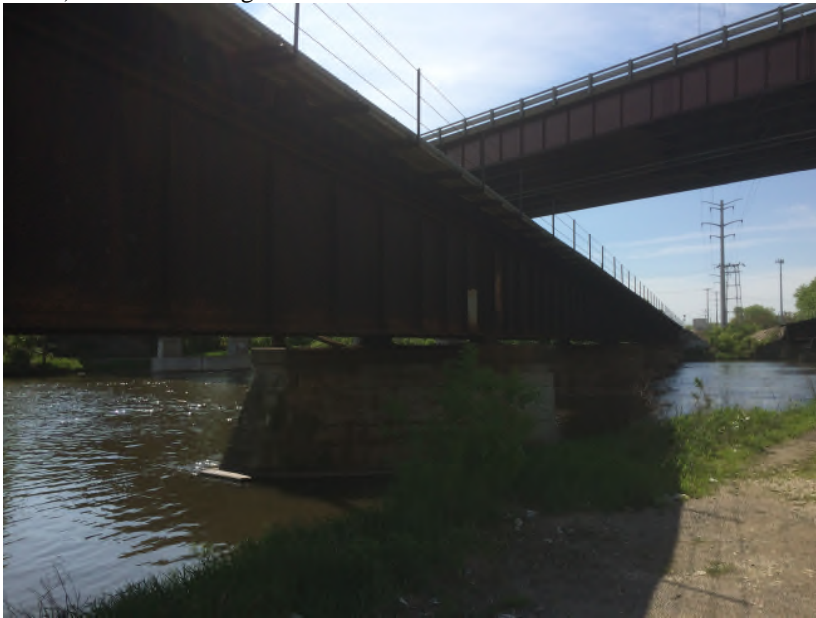
Photo 3: Facing southeast towards the METRA MDW Fox River Bridge.
