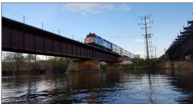
Looking South: Overhead high-tension powerline towers are located in between the two rail bridges.
