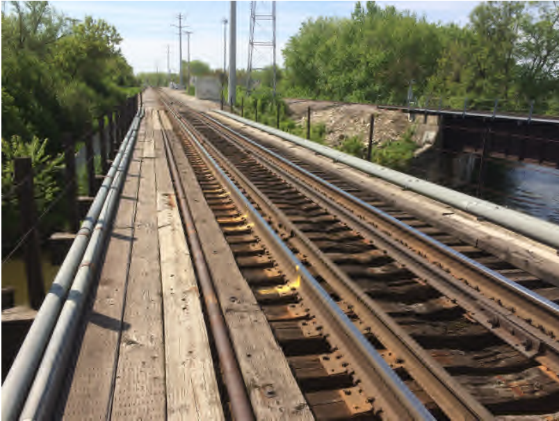
Photo 1: Facing southeast towards the METRA Milwaukee District Westline (MDW) Fox River Bridge.
