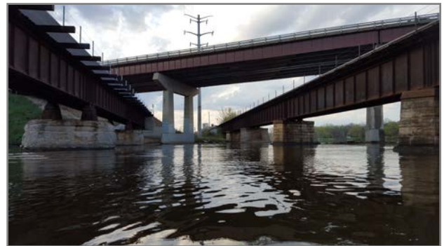
Looking North: The existing Metra bridge is on the right, the UPRR bridge is on the left, with the US Route 20 bridge overhead.
