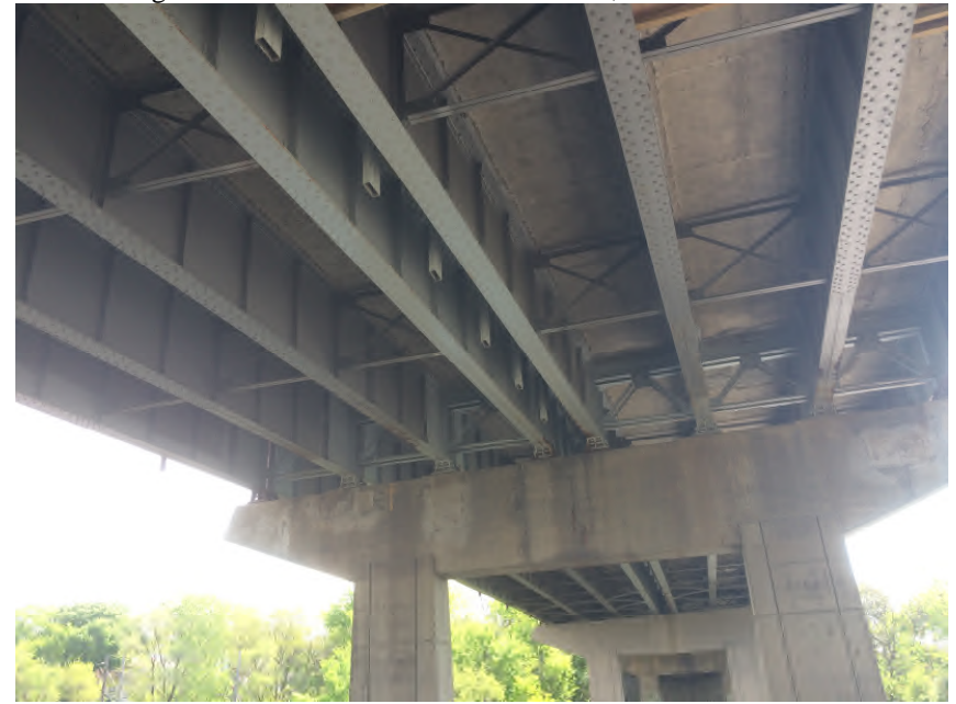
Photo 8: Representative photograph from under the U.S. Route 20 Bridge over the Fox River.
