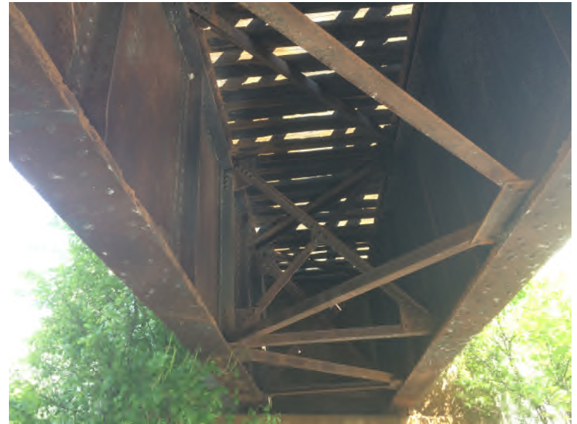
Photo 4: Representative photograph from under the METRA MDW Fox River Bridge.
