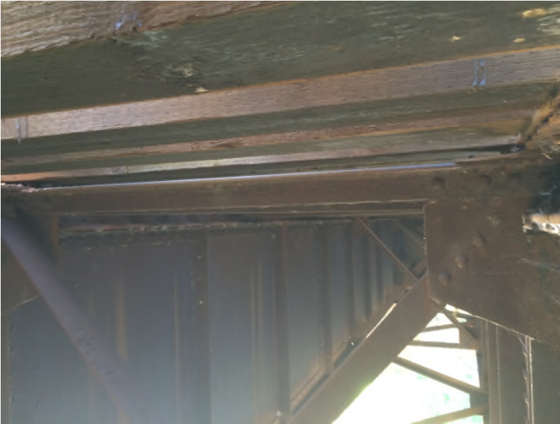
Photo 5: Representative photograph from under the METRA MDW Fox River Bridge.
