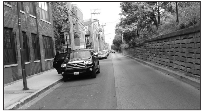
This photo of an area along the UP North right of way on the north side of Chicago shows the existing retaining wall and streetscape.
