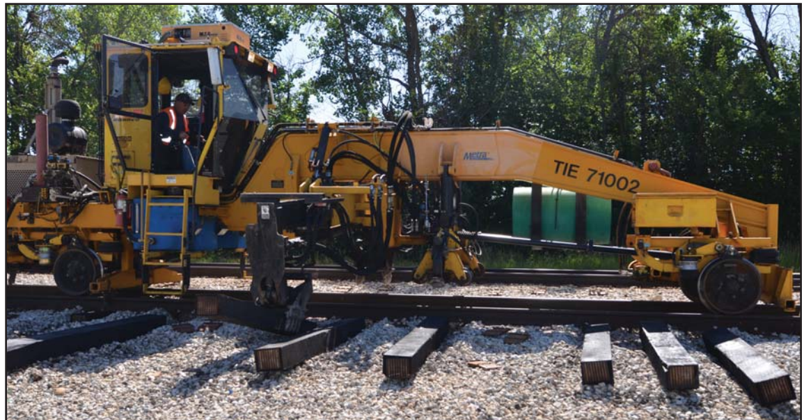
A tie inserter machine places a new tie under both rails as part of a tie replacement project last month.
