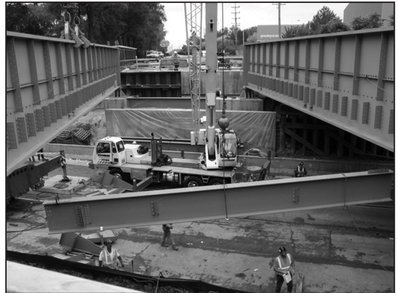
Keeping up with infrastructure improvements, such as last year’s replacement of the Milwaukee North Line bridge over Golf Road, will be difficult without greater funding for our capital budget.
