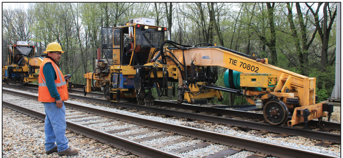
Assistant Track Foreman Benjamin Contreras oversees the replacement of ties on the Rock Island Line near Mokena last month. The machine is a tie inserter that pushes new ties under the rails.
