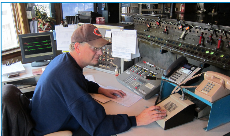
Train Director Dave Reiss communicates with dispatchers and engineers about which trains are about to enter the complex system of switches at Tower A2.
