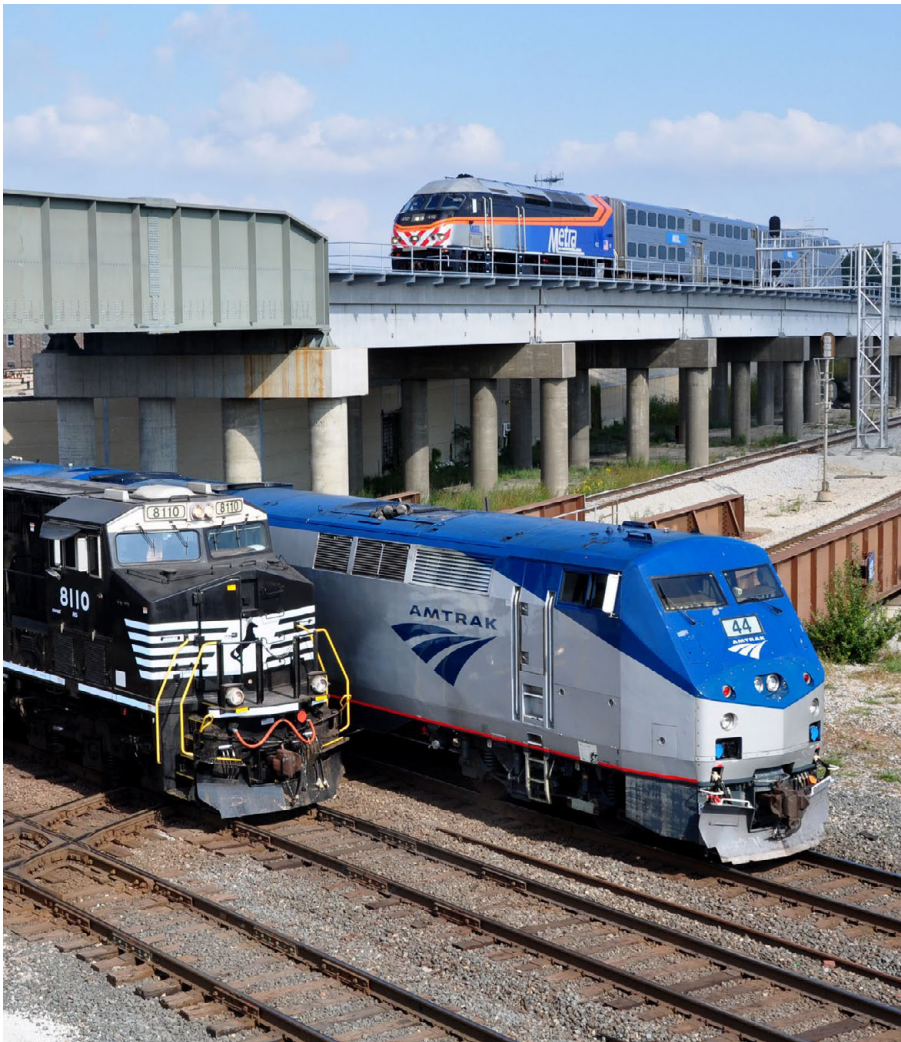
Construction of the Englewood Flyover has eliminated conflicts between RID trains and freight and Amtrak trains at a critical rail junction near 63rd Street in Chicago
