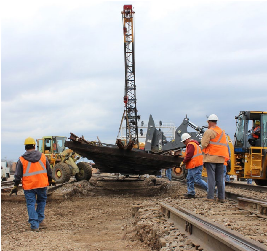
Track work at A-5 Junction in Chicago
